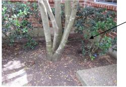
Note: Client is urged to keep soil levels a minimum of 4"-6" below top of slab and graded away to promote positive drainage and to prevent water from ponding around foundation. Proper soil levels will also help detect insects should they try to enter the home from the
